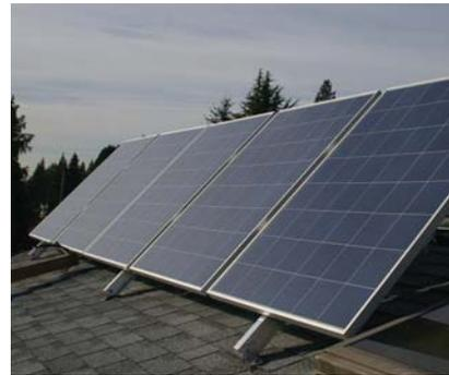
These solar photovoltaic panels are installed on a house in Burnaby. When the panels produce more electricity than is needed by the house, the excess is exported to BC Hydro through net metering.
