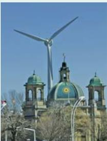
Exhibition Place, on Toronto's waterfront, is host to a 600 kW, 30-storey wind turbine. North America's first urban commercial-scale wind turbine is jointly owned by a local for-profit co-operative (Windshare) and by the City of Toronto's energy utility (Toronto Hydro). The turbine was constructed in 2002, at a total project cost of \$1.8m. It produces around 1000 MWh every year, enough to power approximately 100 homes.
