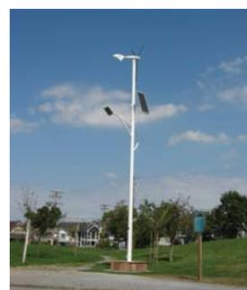
The City of Richmond is testing a new type of lighting system, generating both wind and solar energy, and storing the electricity to a battery to power the street light at night.
