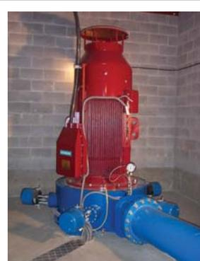
The District of West Vancouver is generating power from its drinking water system, with a 200 kW turbine that replaced a pressure-reducing valve.
