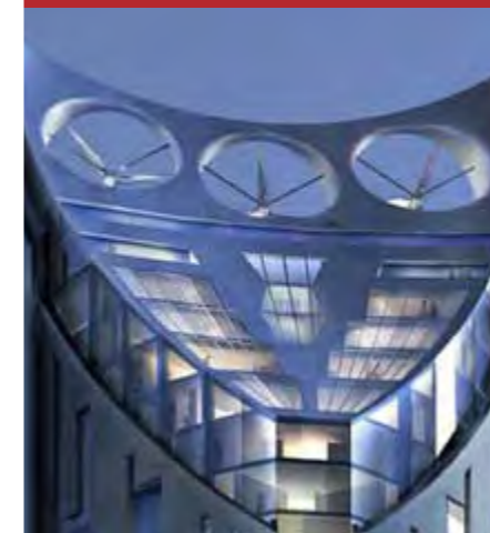
FIGURE 9: RAZOR BUILDING LONDON
