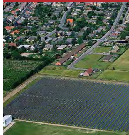
FIGURE 8: MARSTAL DISTRICT HEATING
