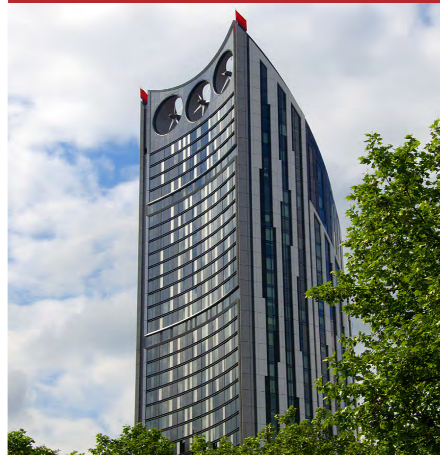
FIGURE 60: STRATA SE1 BUILDING INTEGRATED WIND TURBINES, LONDON, UK SOURCE: SKYSCRAPERCITY
