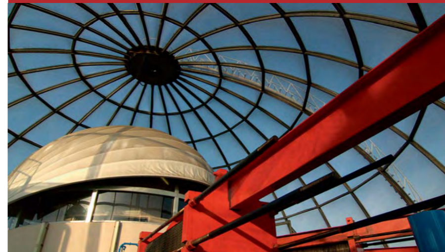
FIGURE 64: MEAUX GEOTHERMAL PLANT, PARIS GEOTHERMAL DISTRICT HEATING NETWORK SOURCE: FRENCH ENVIRONMENT & ENERGY MANAGEMENT AGENCY
