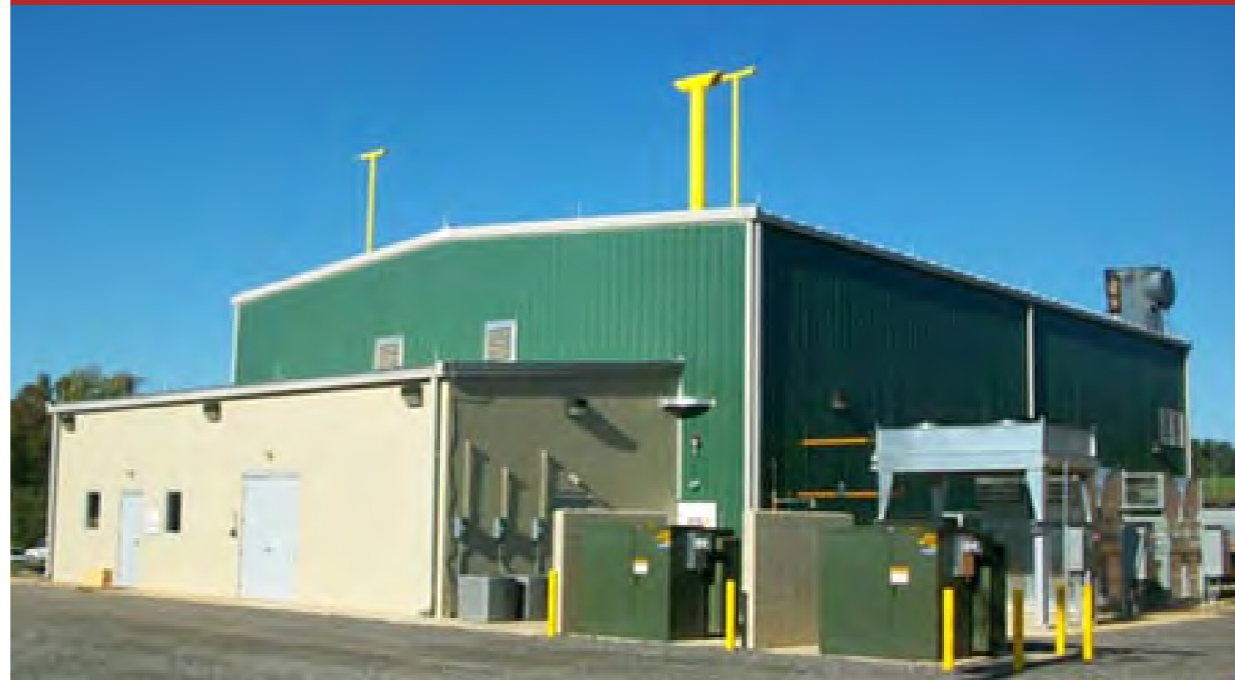
FIGURE 78: MEADOW BRANCH LANDFILL RENEWABLE GAS GRID INJECTION, ATHENS, TENNESSEE, USA SOURCE: RENEWCO
