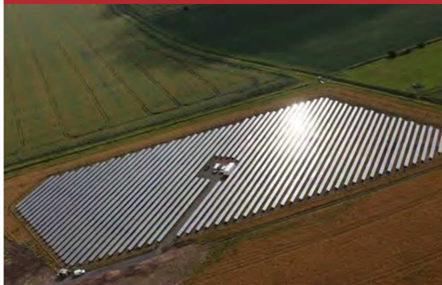
FIGURE 101: FEN FARM SUN PARK, LINCOLNSHIRE, UK (ONE OF THE PROJECTS FUNDED BY ECOBOND ONE) SOURCE: BEBA ENERGY
