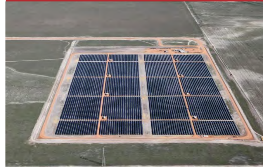
FIGURE 68: GREENOUGH RIVER SOLAR PV FARM, WESTERN AUSTRALIA SOURCE: GREENOUGH RIVER SOLAR FARM
