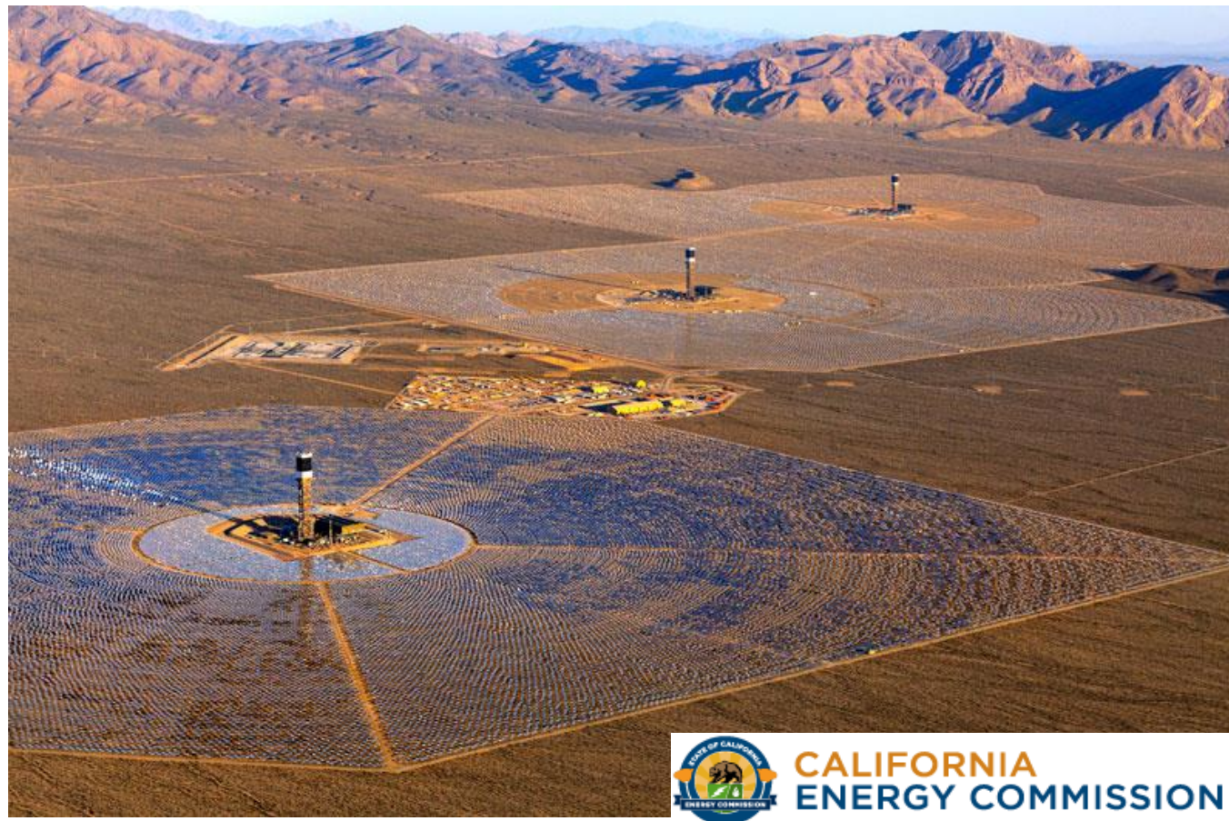
Ivanpah Solar Thermal Station
