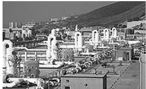
Photo 5: Point Loma Wastewater Treatment Plant
