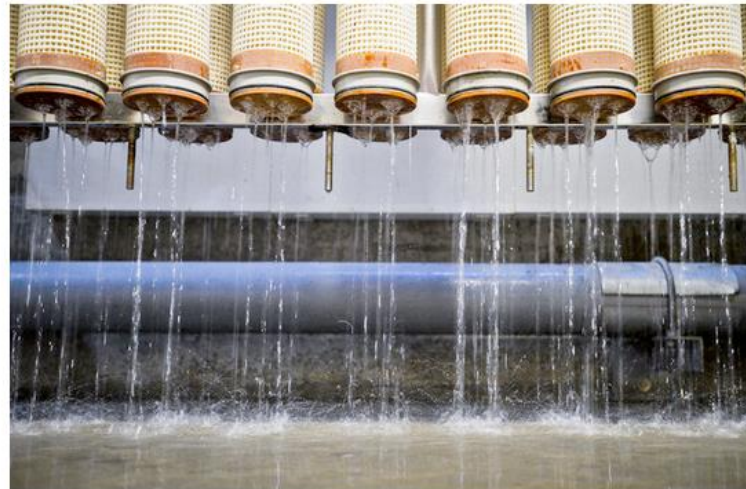
Filtering membranes in an Orange County, Calif., water purification facility. The plant opened in 2008 during the state's last drought. Stuart Palley for The New York Times
